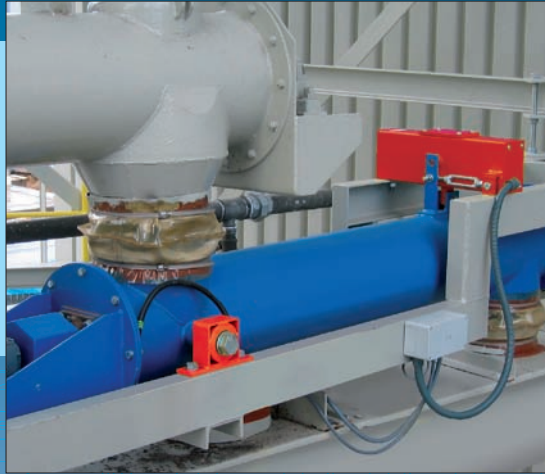
Meetprincipe Impakt flowmeter
